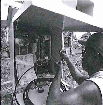
Photo 2: Installation of AHMS in Gizo by SIMS staff
