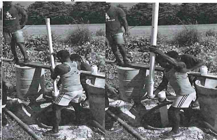
Photo 7: Preparation for well deepening in Taro. Photo 8: Well deepening using simple technology Photo 9: Removal of gravel/sand/mud from the well.
