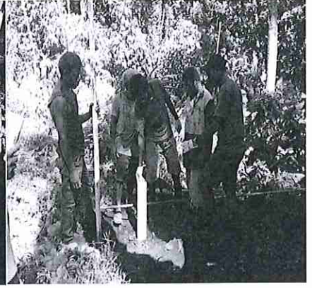
Photo 6: Installation of pipes into the well
